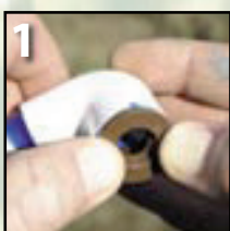
1 Glue brown compression adapter into 1/2" PVC slip fitting
