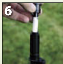
6 Install MP Rotator
