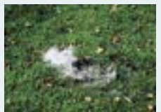
An undetected lateral line rupture is not only wasteful, the flooding can also damage turf and ground cover. If the rupture is on or near a hillside, there can also be erosion damage.
